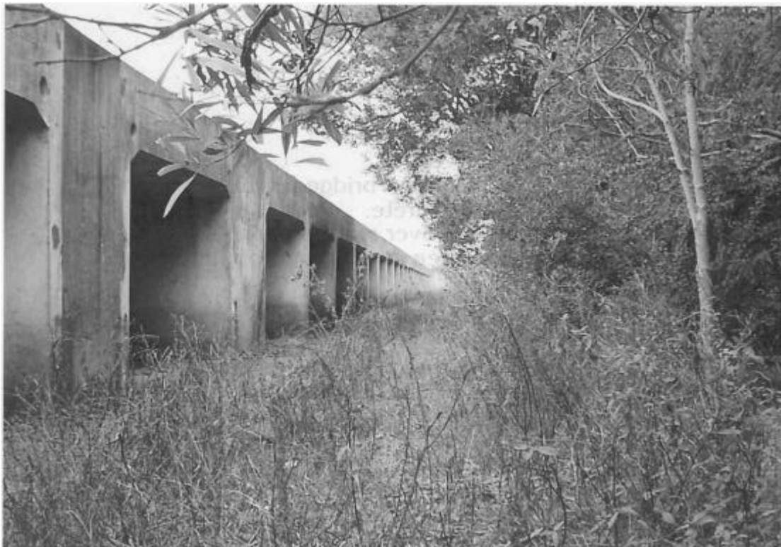
Figure 4.1 A causeway at Tyagarah using several culverts
