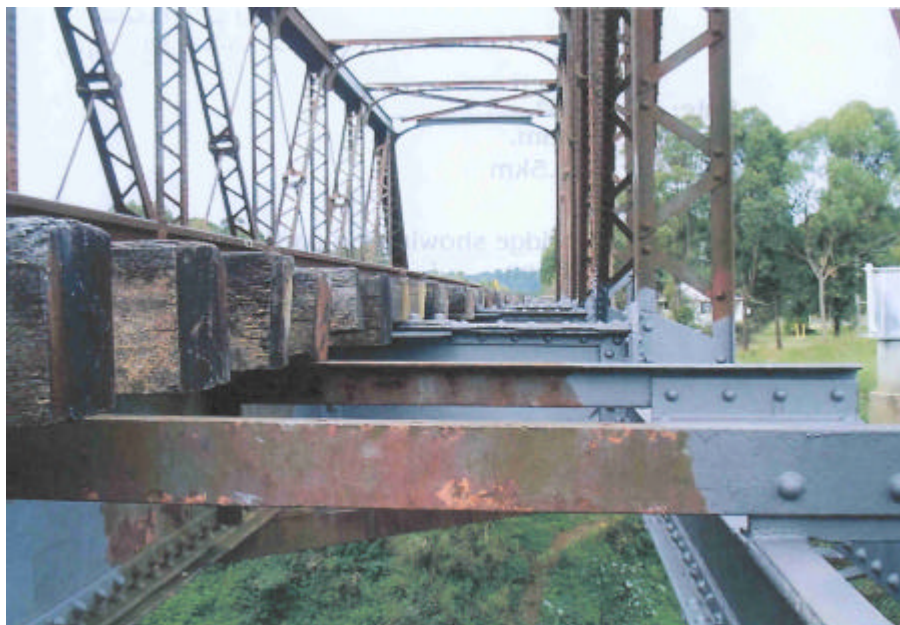
Figure 2.2 The Eltham Bridge
